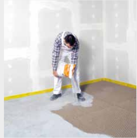
Apply fermacell Honeycomb Infill
