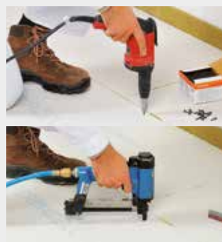
Fix by screwing ... or stapling within 10 minutes - stand on the overlapping edge element
