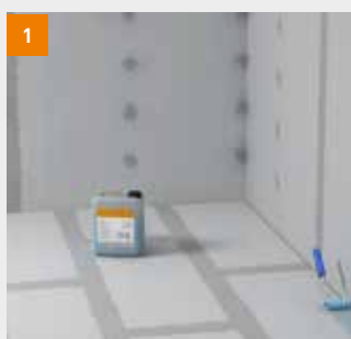
1 Apply fermacell Deep Primer to perimeter wall area ...
