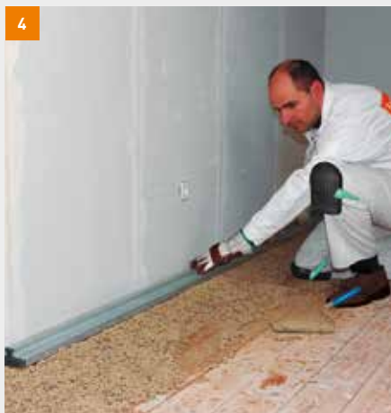
4 The first levelling edge is laid out and aligned
