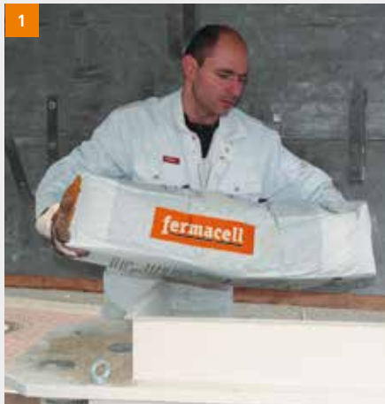
1 Thoroughly mix the entire contents of the bag in a suitable mixer ...
