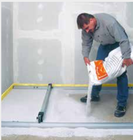
Apply fermacell Levelling Compound
