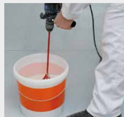
Mix with a suitable mixer at a low speed, until a homogenous, lump-free levelling compound is created
