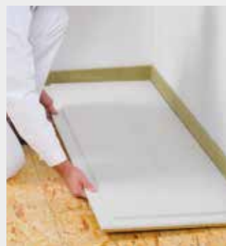
Install the fermacell Flooring Element
