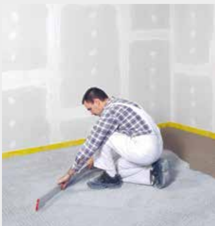
Level out fermacell Honeycomb Infill
