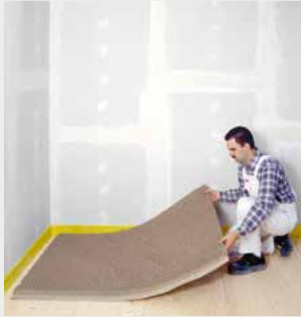
Lay fermacell Honeycomb System
