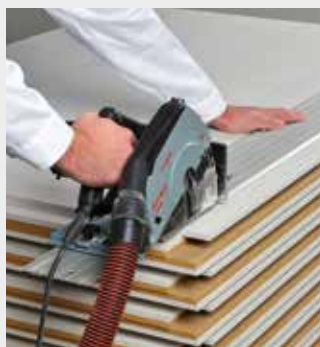
Saw off any protruding edges for the first row
