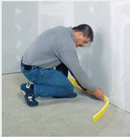
Fitting the perimeter strips
