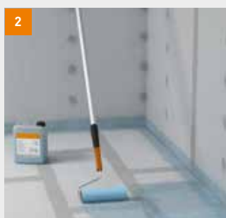
2 ... and floor area using a roller
