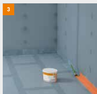
3 Apply fermacell Waterproofing Application to the internal corners
