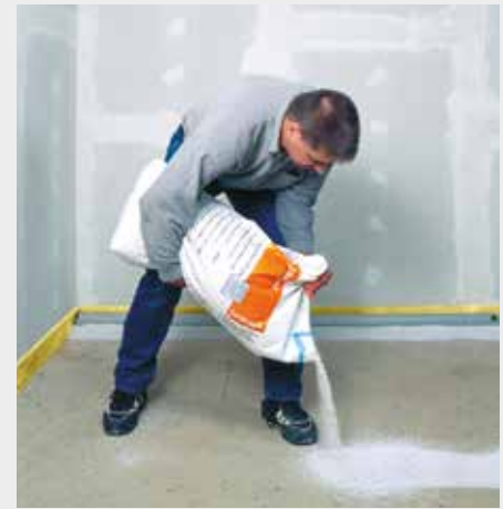
Preparing the area to be levelled
