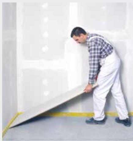
Lay fermacell Flooring Elements
