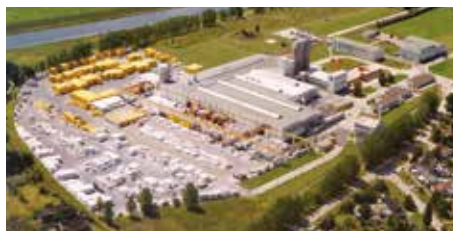
Calbe Factory, Germany
