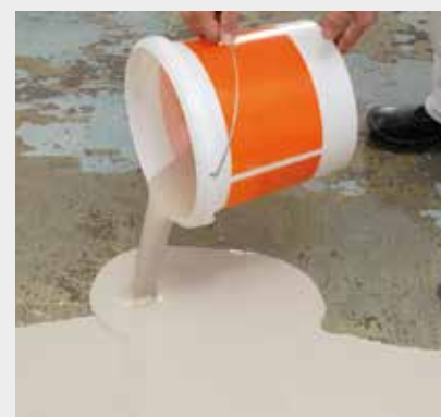
Pour out self-levelling compound and level off
