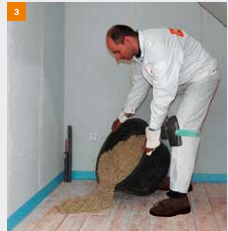
3 The bonded levelling is then laid out as required
