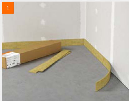
Servalindi paigaldamine.
